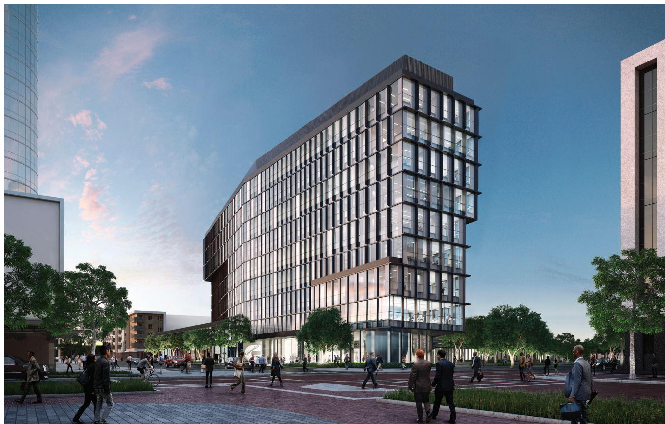
Cummins Indy Distribution Headquarters Indianapolis, Indiana Image credit: Deborah Berke Partners
